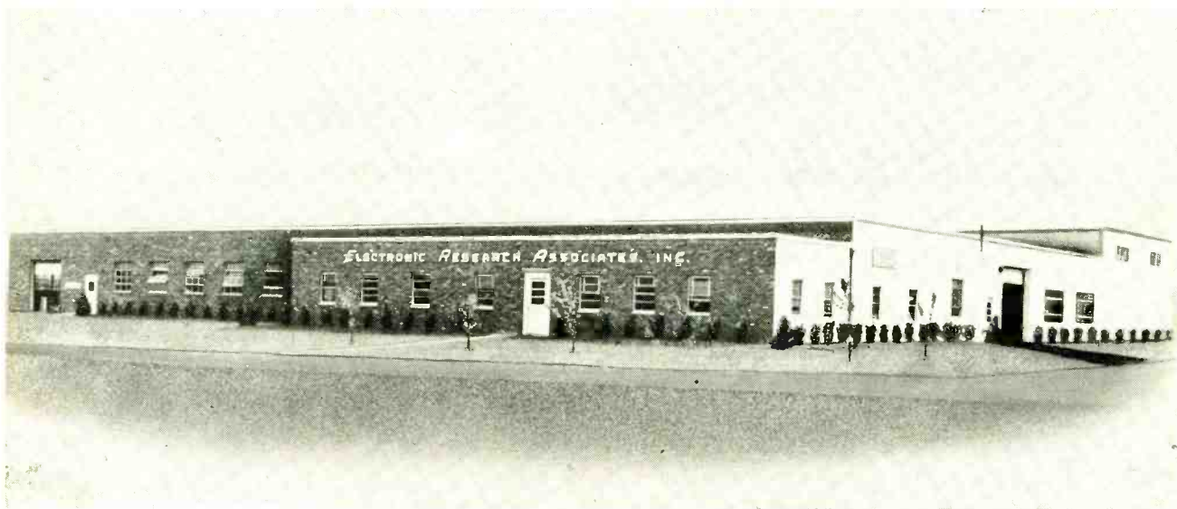
Electronic Research Associates' enlarged facilities
