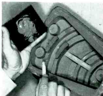
Filling holes in plastic molds. After adhesive is cured, repair can be sanded, smoothed and buffed to gloss finish
