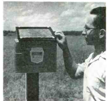
Solar cells mounted on battery case supply power for electric fence
